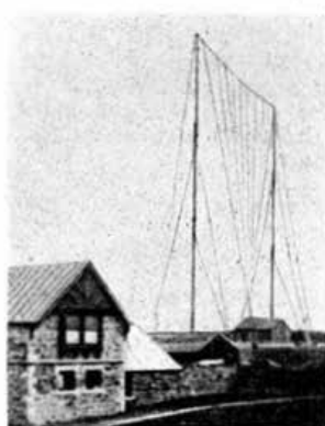
The 170' masts with the 60-wire fan-shaped aerial at Poldhu, used for Marconi's first transatlantic experiment in 1901.
