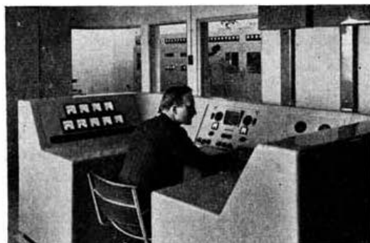
The control desk for the vision and sound transmitters. The control room has windows overlooking the transmitter hall so that the engineer on duty can see the transmitters.
