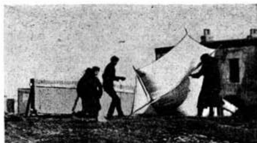
Preparing the kite which supported the aerial on which the first transatlantic signals were received in Newfoundland.
